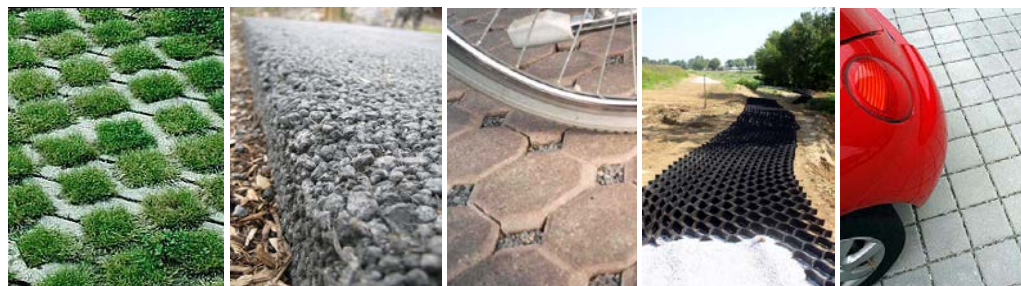
(a) Reinforced Turf Concrete Grid Paver Driveway (Source: www.buildinggreentv.com ) (b) Porous Asphalt Roadway/Path (Source: creativeconcrete4you.com ) (c) Concrete Permeable Paver Plaza (Source: http://www.uni-groupusa.org/ ) (d) Reinforced Gravel Trail (Source: http://www.ia.nrcs.usda.gov ) (e) Concrete Permeable Paver Patio (Source: http://www.uni-groupusa.org/ )
