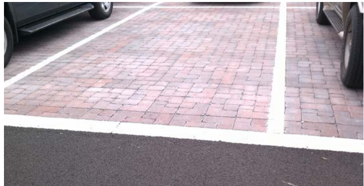
Figure 3 Parking Lot Permeable Concrete Pavers
