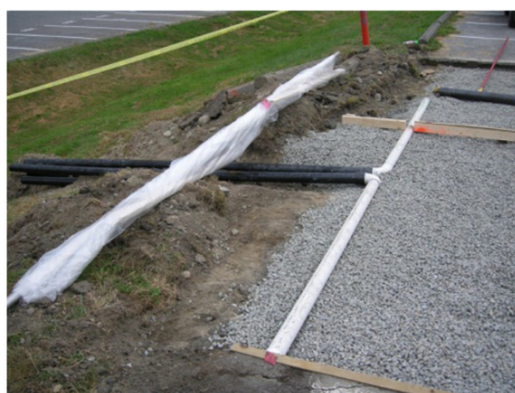
Photo 2. Perforated pipes on top of crush connecting to ABS pipes.
