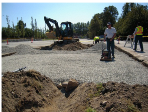
Photo 4. Compaction of clear crush and simultaneous excavation.
