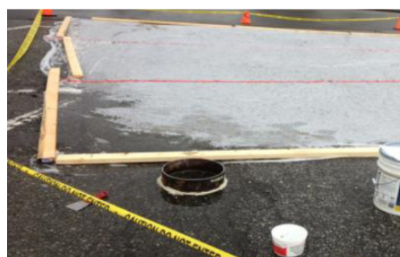
Photo 11. Ring used for the in-place percolation test.
