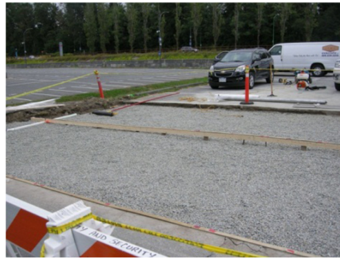
Photo 5. Compacted crush ready to receive pervious concrete.
