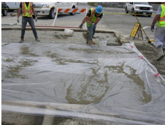
Photo 8. Finished concrete slab (Bay 1) covered with polyethylene sheet.
