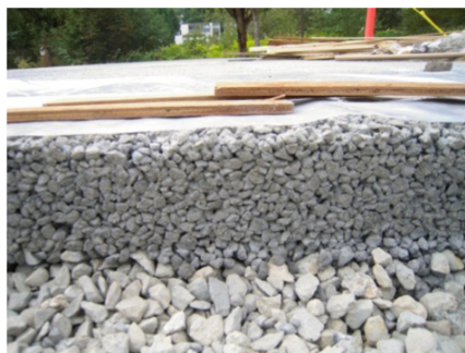
Photo 9. Pervious concrete cross-section after saw cut.
