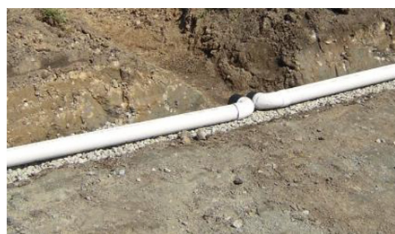
Photo 1. Perforated pipes above the subgrade.
