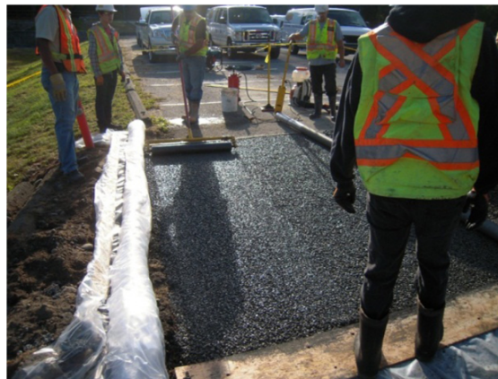
Photo 7. The second roller giving the desired finish of the concrete.
