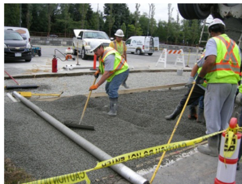
Photo 6. Roller screed and leveling of pervious concrete.
