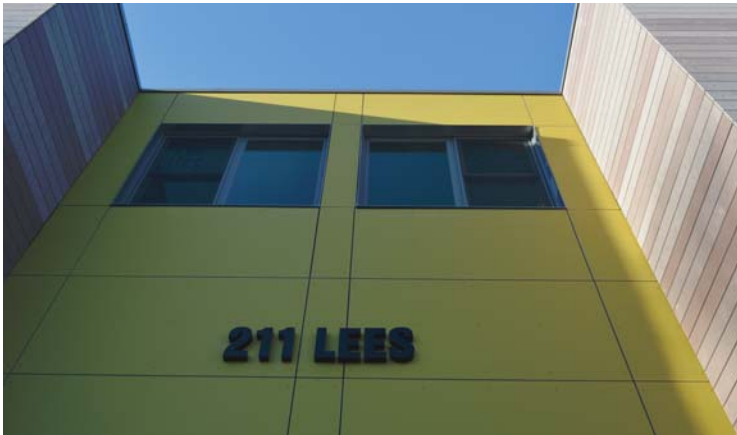
Redevelopment at a Lees Avenue housing complex following a devastating fire in 2013. (Credit: Ottawa Community Housing)
